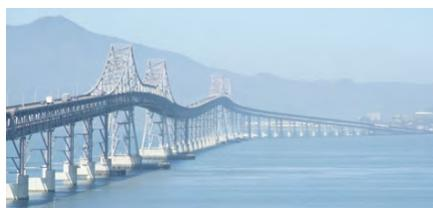
BATA plans to request bids in Spring 2017 for Package B to convert the top deck shoulder into a barrier-separated, ten-foot wide, bidirectional Bay Trail for use by both pedestrians and cyclists traveling between Richmond and San Rafael. Both the Point Molate and bridge Bay Trail sections are scheduled for completion in Spring 2018.
